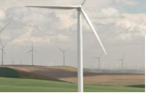
Wheat Field consists of 46 Suzlon S88 2.1MW wind turbines.
