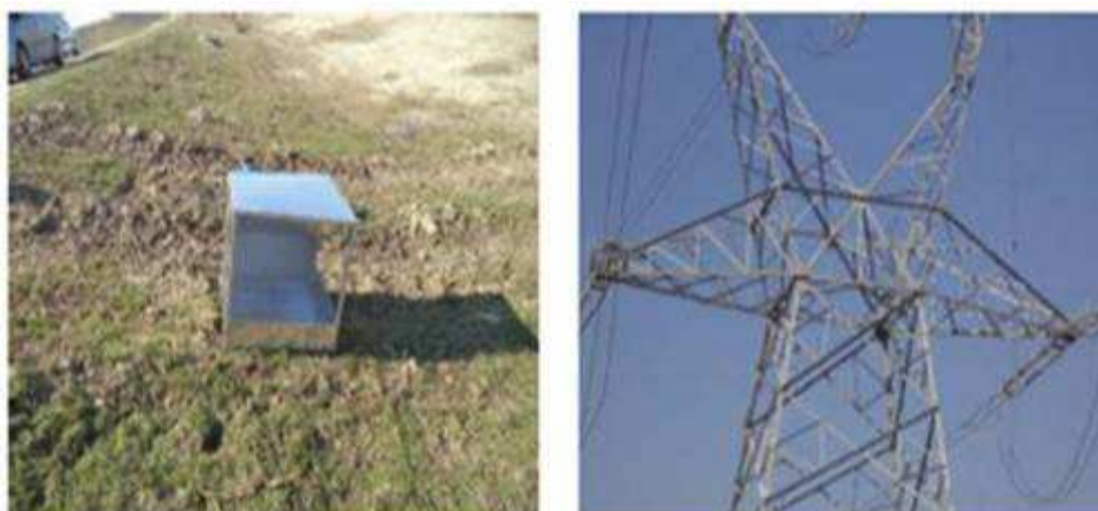
Figure 6. Artificial nests installed on the high voltage poles
