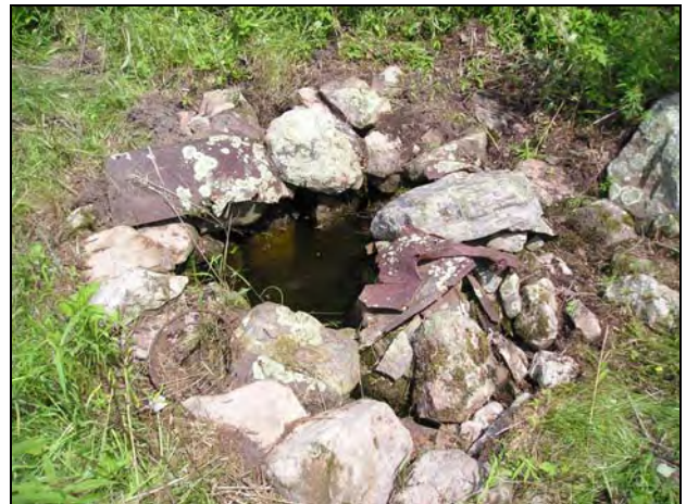
Large 7-foot-diameter stone-lined well located at the southwest corner of the barn foundation (view to the east).
