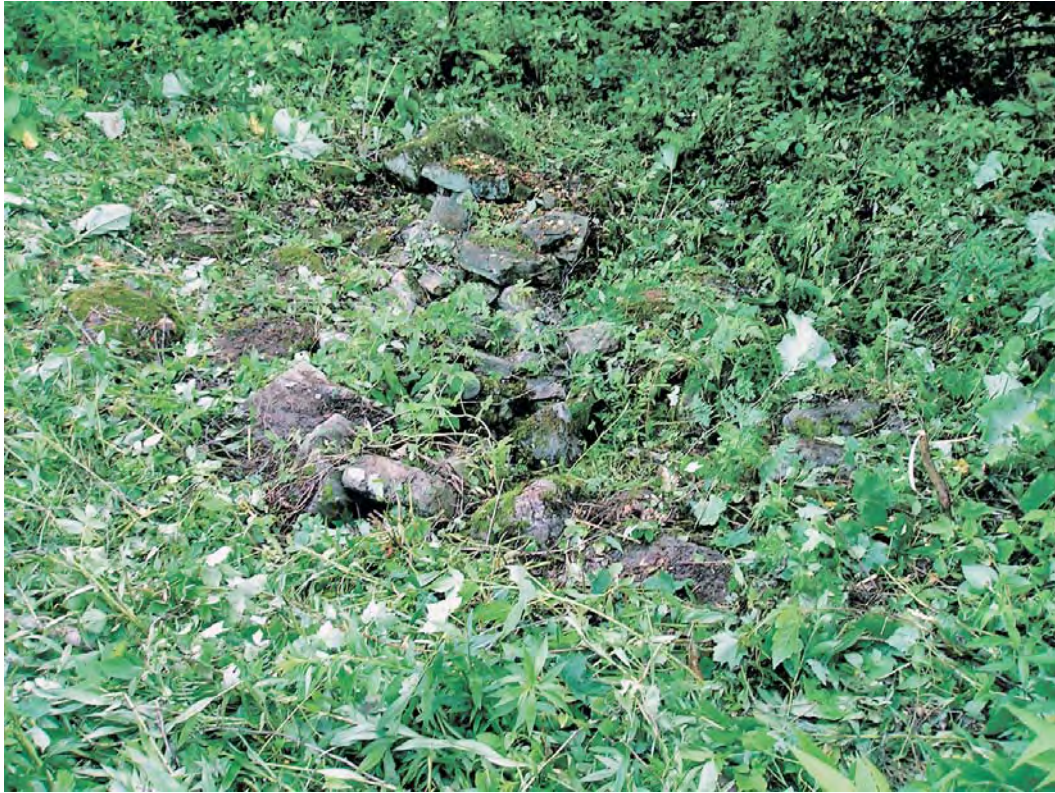
Photograph 25. Pushed-in house foundation or cellar hole at the Wilkins Road Site (OPRHP Site 01907.000087); view to the east.
