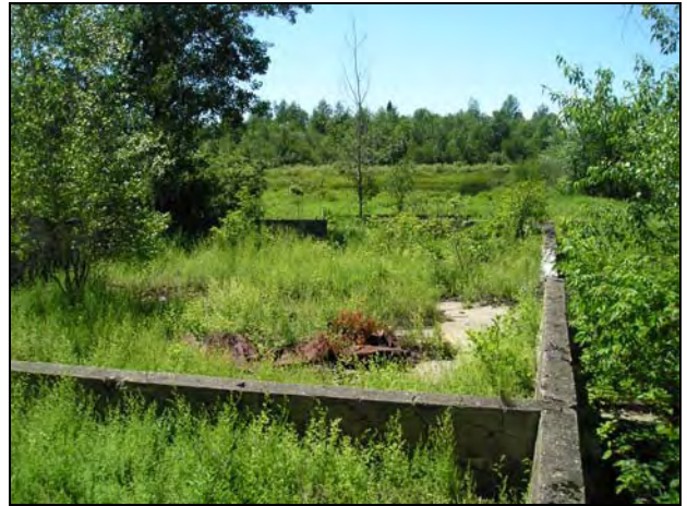
Cement foundation remains of the millworks at Clinton Mills (view west).
