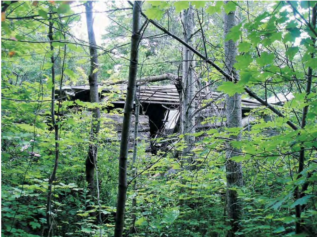
Photograph 35. Existing conditions at the Patnode Road 2 Site (OPRHP Site 01909.000046); view to the southeast.
