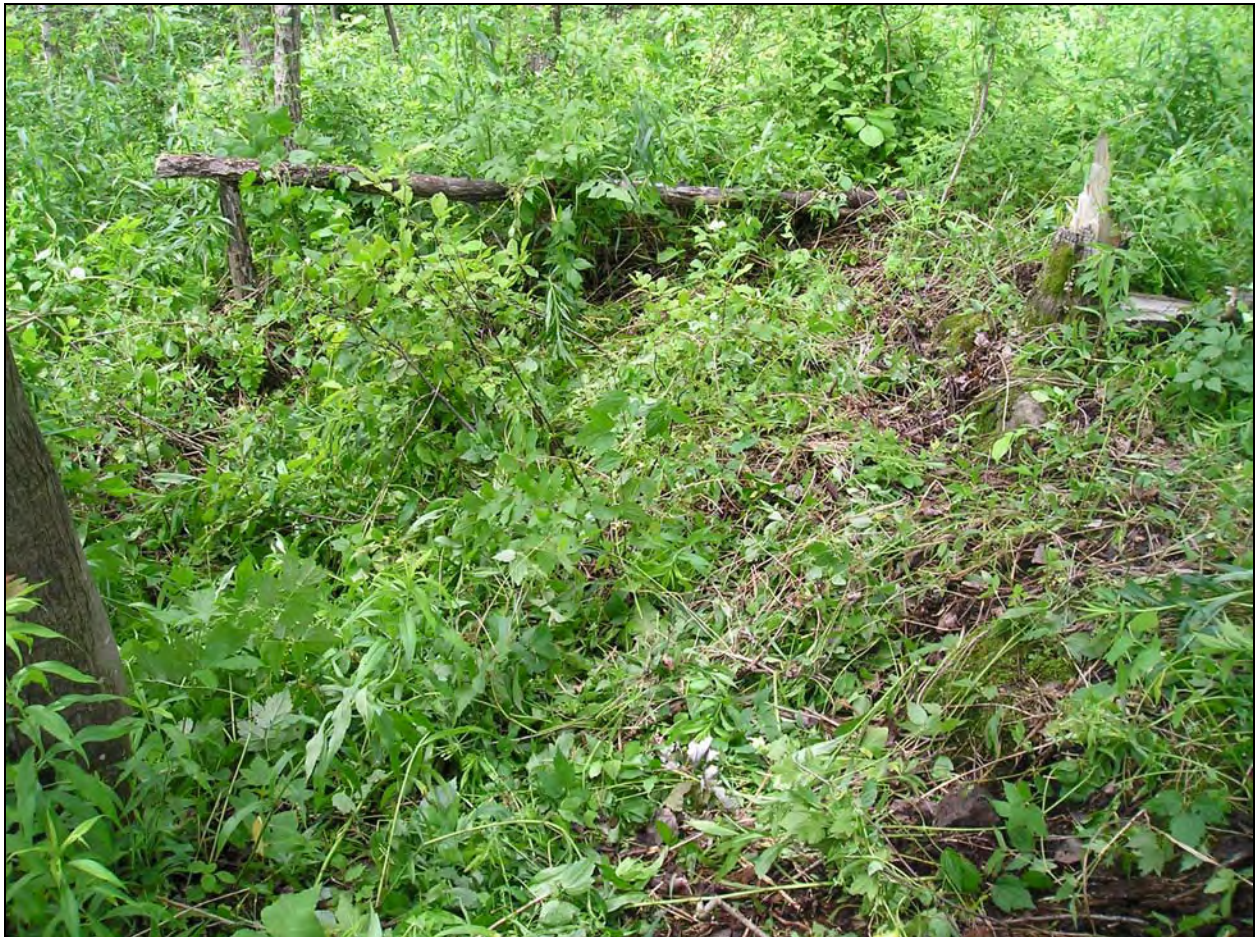
Heavily overgrown foundation remains at the Boomhower & Humphrey Site (view to the north).
