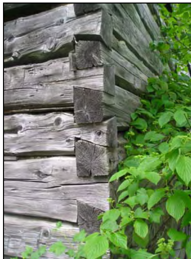
Context and setting of the Patnode Road Historic Site 1 (above); detail of dove-tail construction on the collapsing rough-hewn log house (below).
