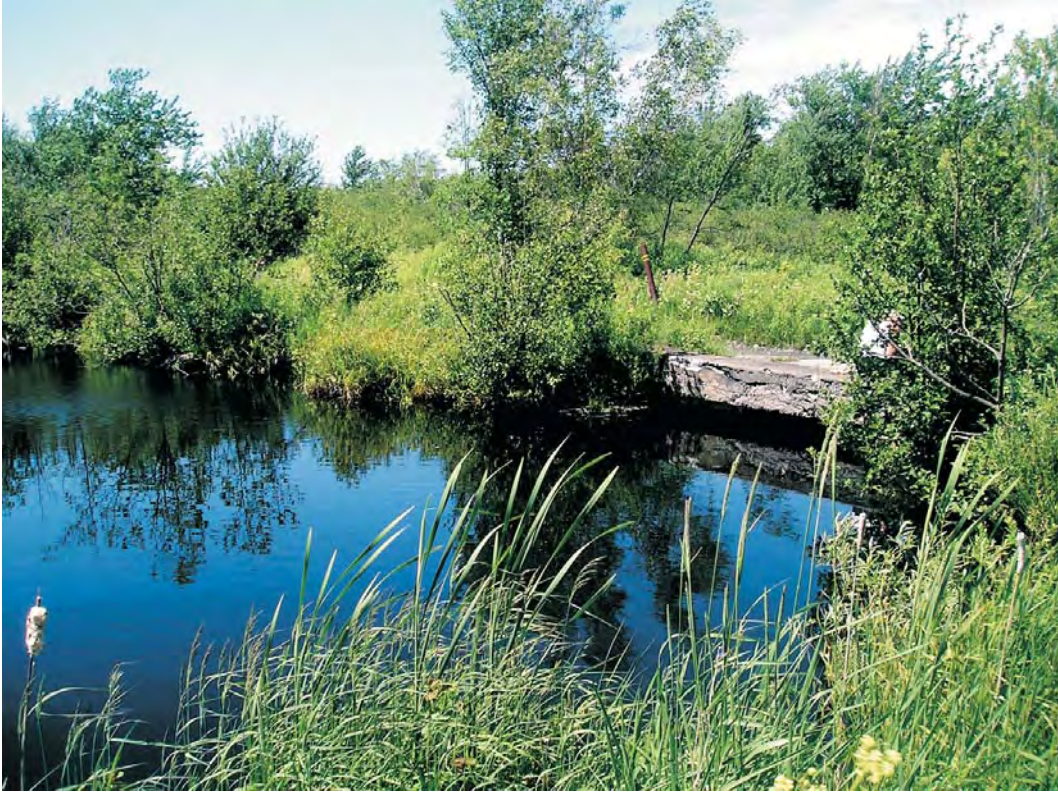
Photograph 19. Dam and millpond along the English River at Clinton Mills (OPRHP Site 01907.000088); view to the west.
