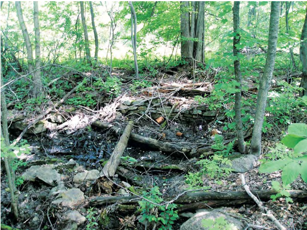
Photograph 30. Foundation remains at the Clark Site (OPRHP Site 01907.000085); view to the south.
