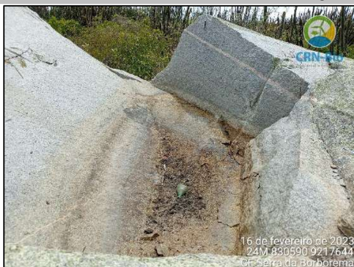
Tanque artificial - P06
