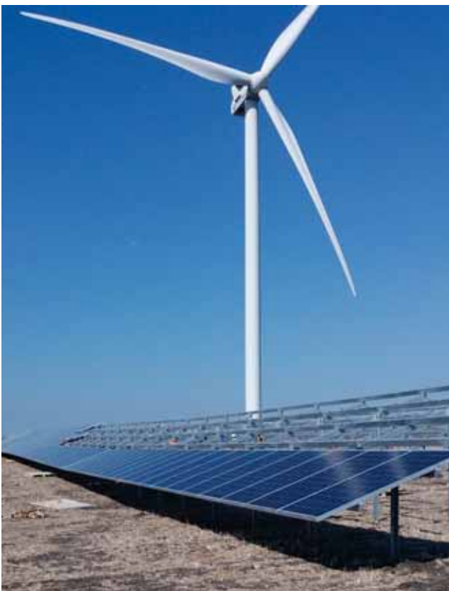
El Conilete hybrid power plant installation
