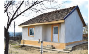
Before and after rehabilitation
