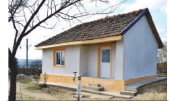
Before and after rehabilitation
